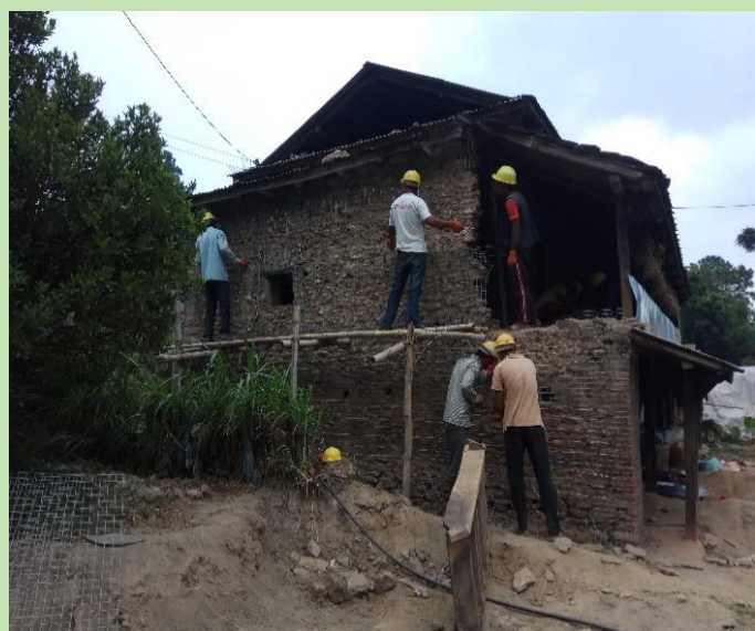
Retrofitting undergoing in Manilal's house
